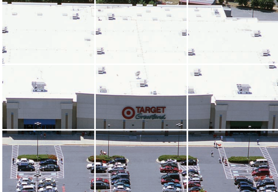
Retailing giant Target Corporation is minimizing its "environmental footprint." Towards that end, the corporation worked with Sika Sarnafil to recycle their old PVC vinyl roof in Silver Spring, MD while installing a new Sarnafil membrane.
